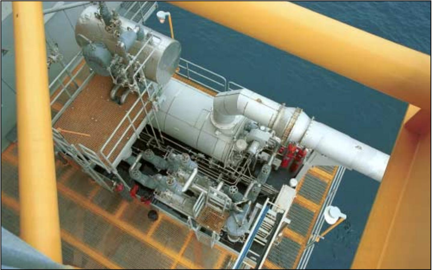
Heatec 5 million Btu/hour heater system on Hickory offshore platform
