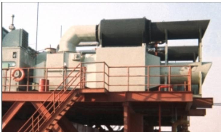
Photo at top of page shows the offshore platform with the two Heatec waste heat recovery units. Closeup photo above shows two of the exhaust stacks that include silencers (the black ones) and one of the Heatec units with its exhaust stack.
