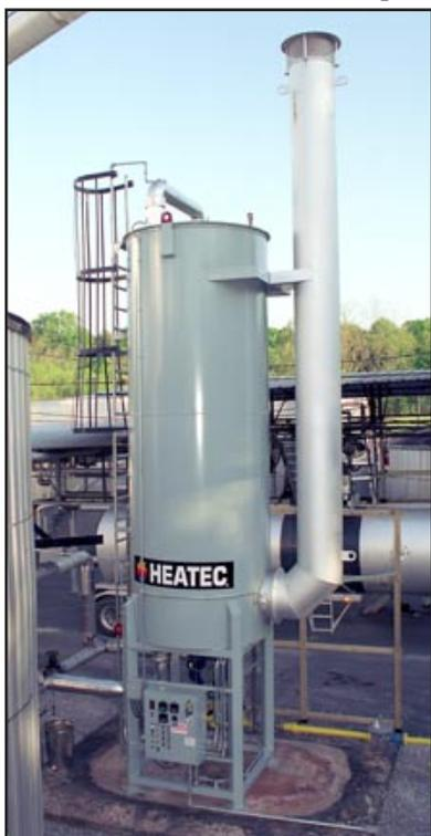
Heatec 5 million Btu/hour helical coil heater
