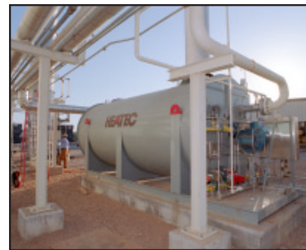
One of two Heatec 6010-50-G heaters at the Bridgeport Gas Processing Plant.
