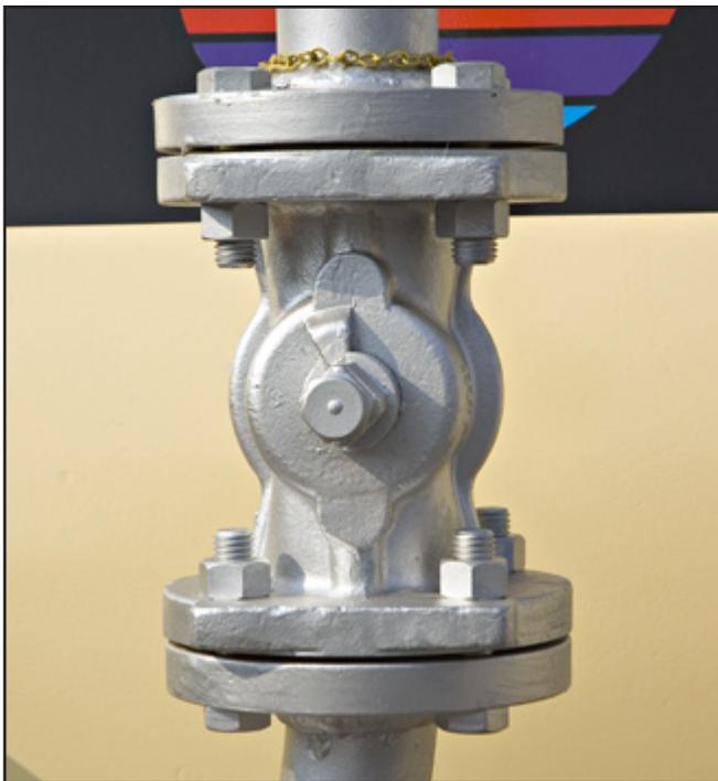
Figure 1. Typical flanged joints used in piping.
