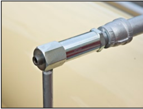
Figure 10. Pressure relief valve used on current preheaters.
