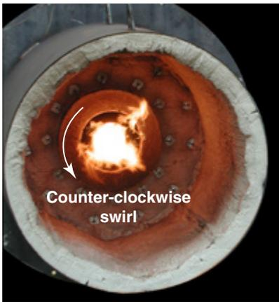
flame pattern, when viewed through the sight glass on the heater end plate should have a counter-clockwise swirl. The flame should be no longer than 1/3 the length of the coil. Flame diameter should be
