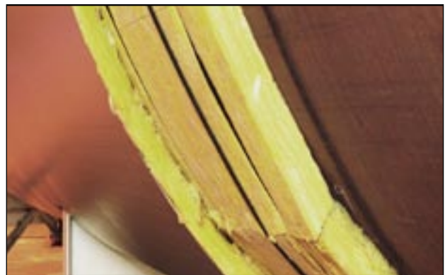
Figure 4. Heatec tanks have 6-inches of Owens Corning fiberglass insulation on sides (2 layers of 3-inches).
