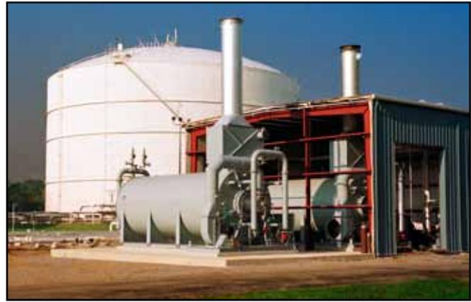
Two 60 million Btu/hour Heatec heaters convert LNG into natural gas for pipeline distribution at this gas plant in Chattanooga, TN. LNG is stored in the large white tank in the background.
