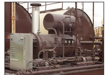
Heatec offers a digital control panel that replaces UE controllers. The panel, called the UE conversion panel, can be mounted at a more convenient location, away from hot oil pipes. And since the controllers are digital, they do not require calibration. For more info, call the Heatec parts department at 1-800-235-5200.
