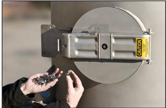
Figure 2. Checking packing for calcium buildup.
