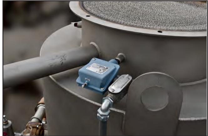
Figure 11. High flue gas temperature switch.
