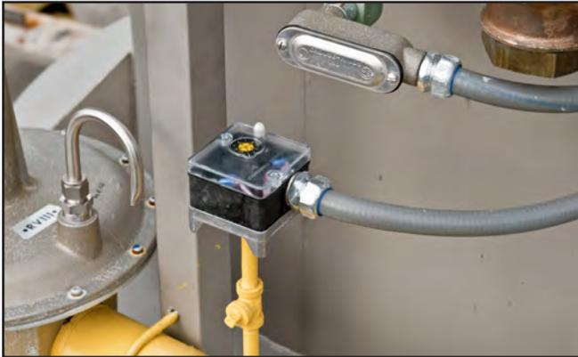
Figure 10. Low fuel gas pressure switch.
