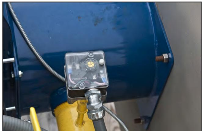
Figure 9. High fuel gas pressure switch.
