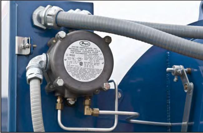
Figure 14. Low combustion air switch.
