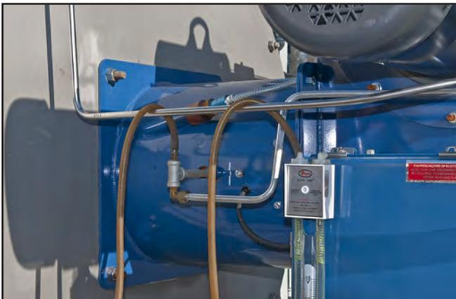
Figure 8. Manometer connected to tee at pilot gas line.
