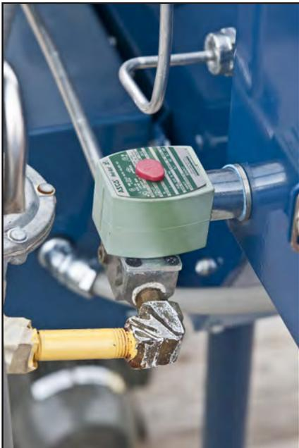
Figure 12. Gas pilot solenoid.
