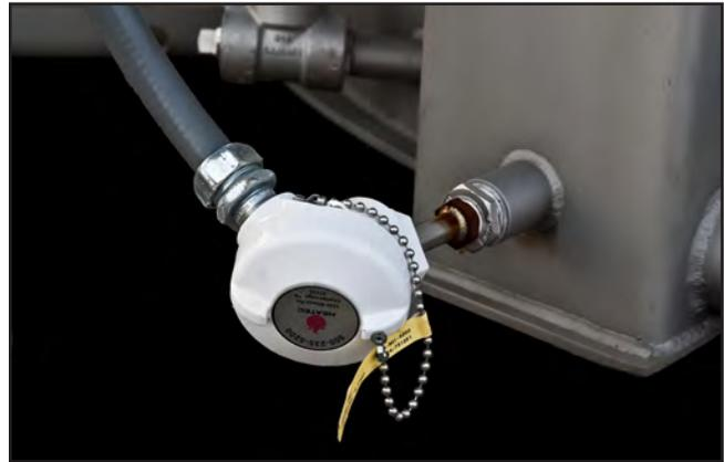
Figure 6. Thermocouple in reservoir at bottom of heater.
