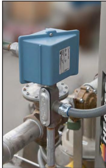
Figure 13. Inlet water pressure switch.
