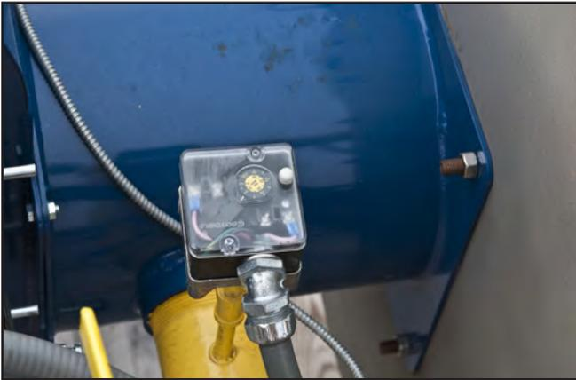
Figure 8. High fuel gas pressure switch.
