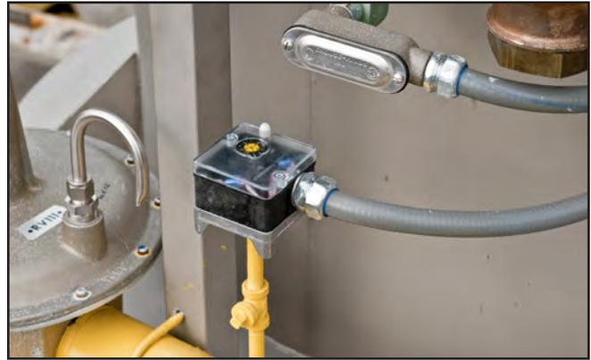
Figure 9. Low fuel gas pressure switch.
