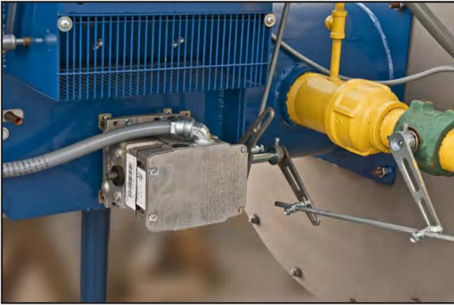
Figure 7. Modulating actuator.
