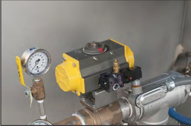
Figure 14. Pneumatically actuated automatic outlet water valve.
