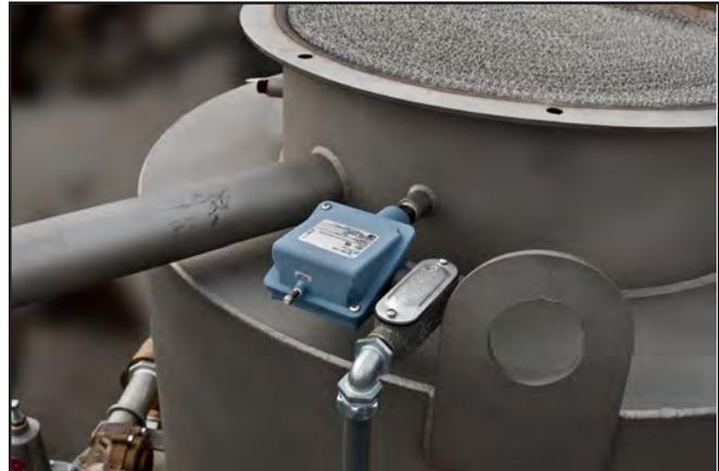
Figure 10. High flue gas temperature switch.
