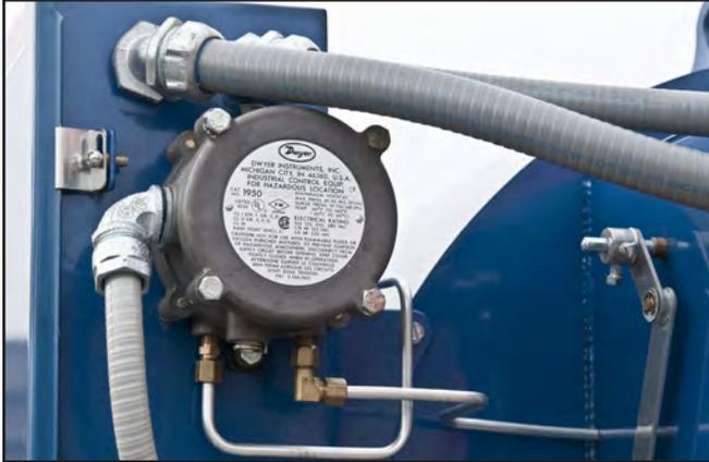
Figure 11. Low combustion air switch.
