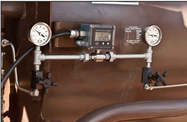
Figure 3. DP switch 4W3A01 installed on a Heatec heater.
