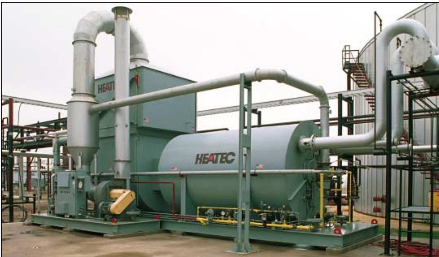
Heatec incinerator system has a combustion chamber (center), secondary heat exchanger (left of center), combustion air preheater (far left) and exhaust blower (lower left.)
