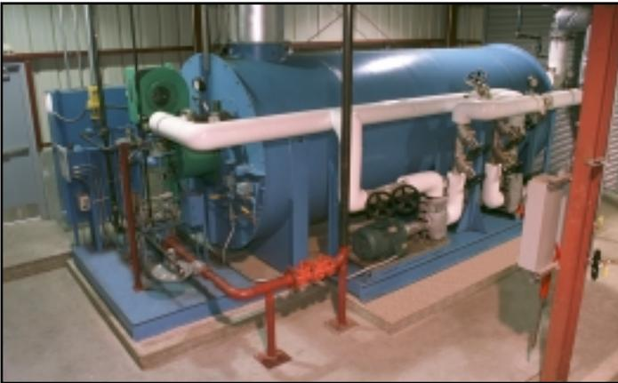
Heatec thermal fluid heater provides process heat for production of polyaspartate polymer
