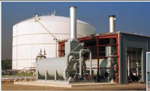
A new Heatec heater (in the foreground) is being installed at the Chattanooga Gas Company. The building that presently houses their first Heatec heater will be extended to enclose both heaters. The heaters convert liquefied natural gas, stored in the large white tank (in the background) to natural gas.
