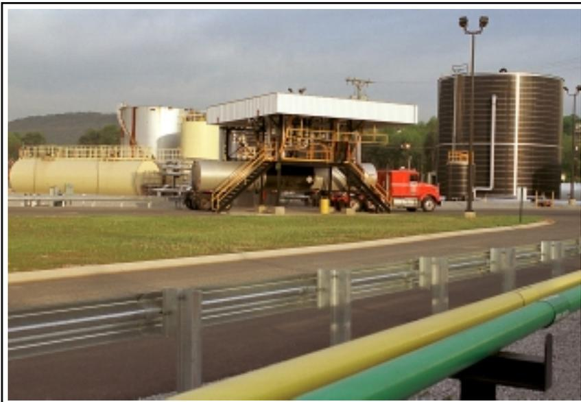
Asphalt tanker receives liquid asphalt for delivery to hot mix asphalt plants. Heatec polymer blending equipment is visible in the background, on the left side of the picture. A 500,000-gallon asphalt storage tank appears in the background, on the right side of the picture.
