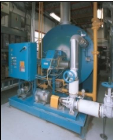
This is the Heatec helical coil heater at the McAsphalt terminal in Toronto, Ontario. It was installed in 1989 and is more than 10 years old.
