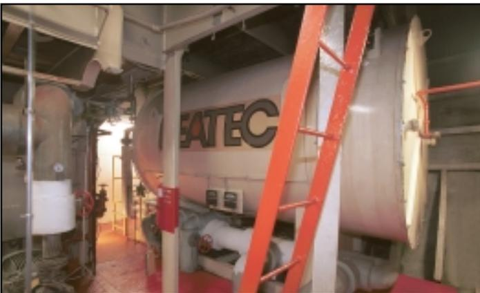
Heatec helical coil heater installed below deck on the McAsphalt barge. It has been in use since 1991 and is more than 9 years old. A long-life coil is extremely important where gaining access for replacement is a major undertaking.
