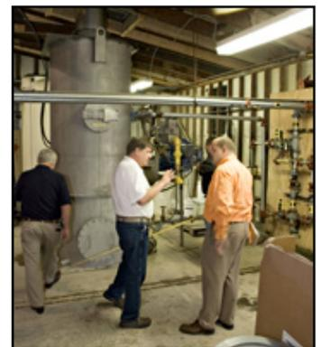
IMI's Monte Larimore (center) speaks with a Heatec representative. In the background is the Firestorm heater with its upper access hatch and lower manway, both for internal cleaning and maintenance.
