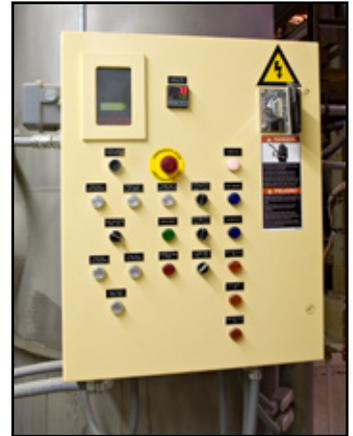
Control panel includes digital controller to set water temperature.
