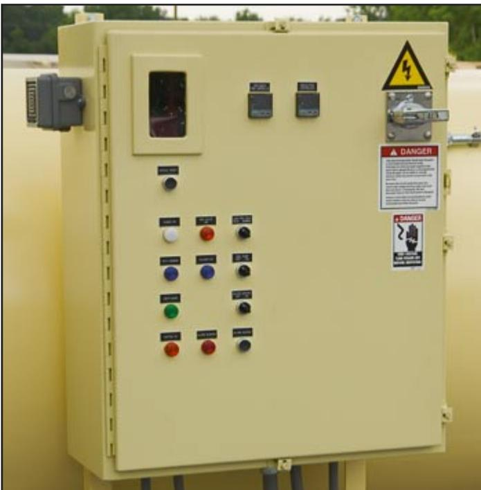
The heater control panel provides protection against water and dust. The Fireeye Flame monitor inside the panel is visible through the glass window. Both the modulating controller and a high media temperature controller are Yokogawa, 1/16 DIN. A laminated wiring diagram is provided inside the panel.
