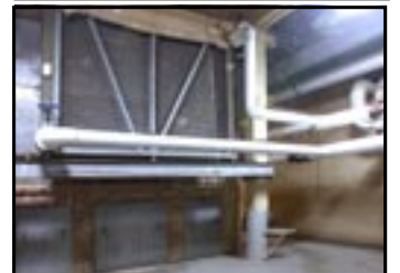
Air passes through large heat exchangers (lower photo), then upward through drying rooms (upper photo).
