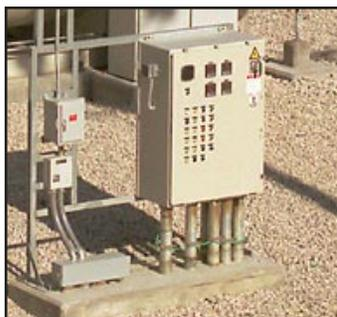
Remotely mounted control panel
