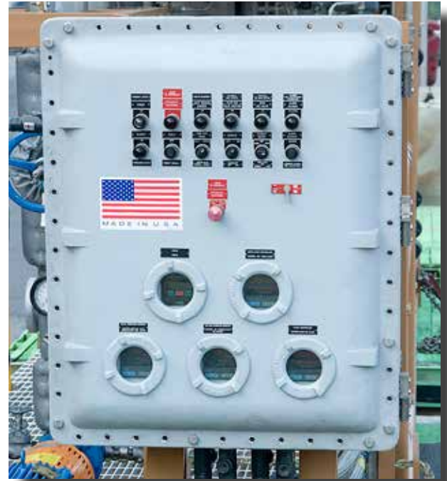
A typical NEMA Type 7 panel suitable for Class I, Division 1 areas. These panels can also be used for Class I, Division 2 areas to eliminate the need for purging.
